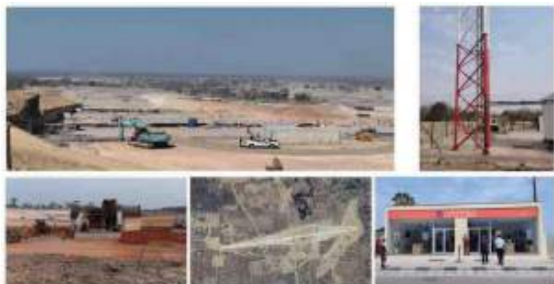
Angola Ndúe Dam Construction Site
