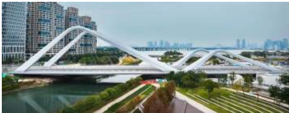
Guiwan River Bridge Project After Construction
